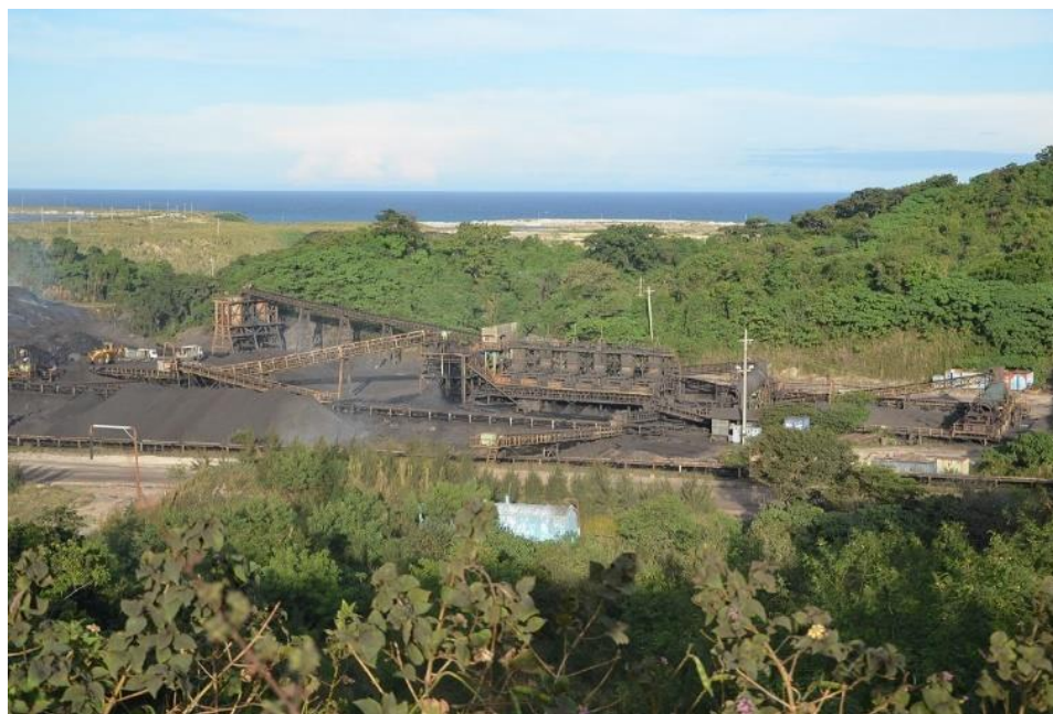
Figure 14. The coal washing plant viewed from the west. (Source: GPPamintuan)
